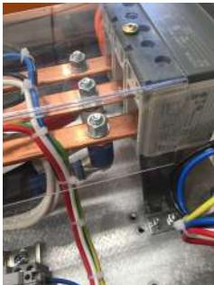
**E-FE-POST** used to provide tap-off for second chassis
